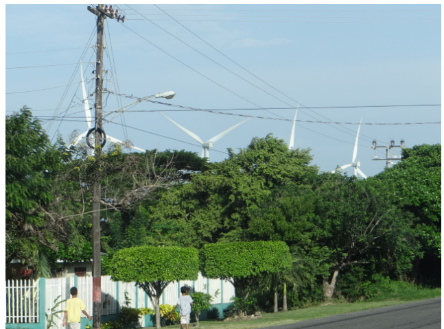
Windenergie in Rivas
