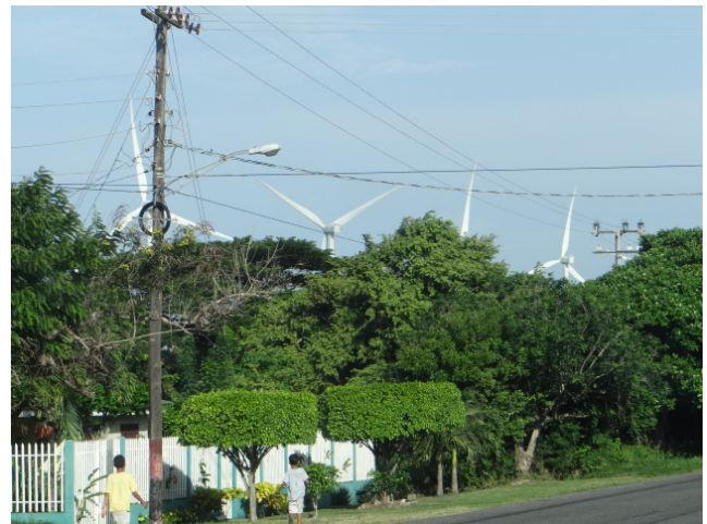
Windenergie in Rivas
